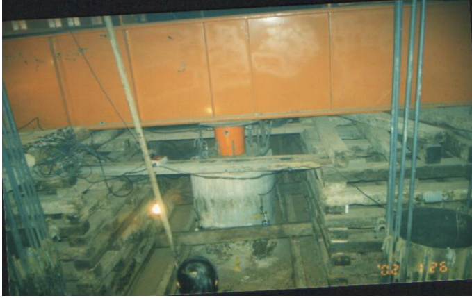
Figure 4. Field pile loading test.
